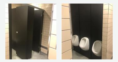
Our made to measure metal framed washroom panelling system, Frameduct, was specified in matching Noir HPL for the WCs and urinals. With Frameduct, all duct space is concealed and can be accessed by opening the secure access panels that are on 90° linear bearing hinges - this makes for simple ongoing maintenance.
